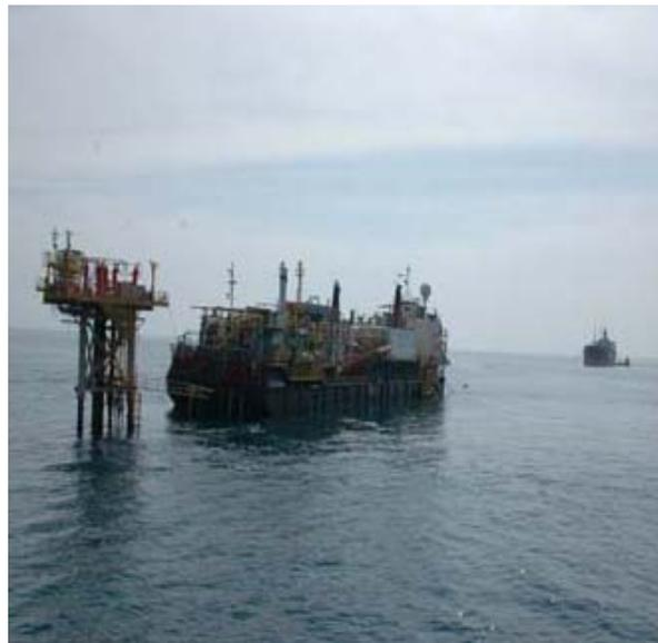
**Well head platform and production barge with storage tanker in background.**
